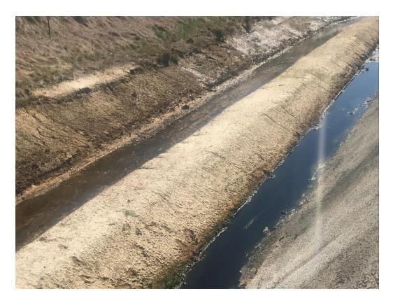
$\label{lem:lemmage} \mbox{Image 3-Perimeter swale to the basin and overflow swale to the discharge point.}$
