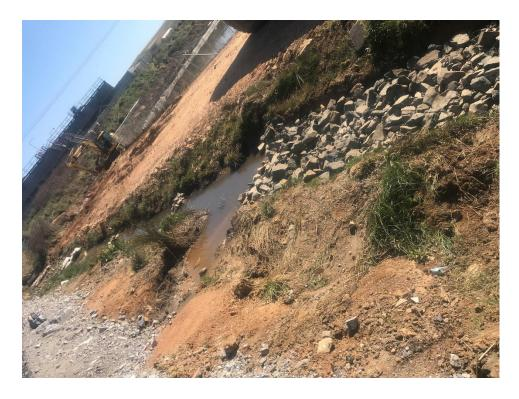
Image 1: Swale drain lined with scour rock
