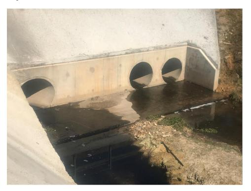
Image 2 – Pipe culvert outlet (showing the internal flow (left) and inflows from adjacent site
